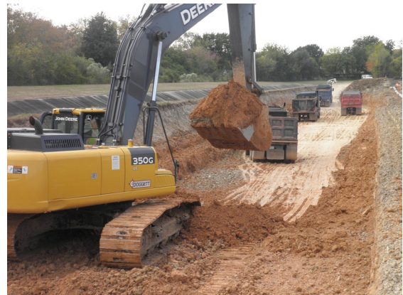
Construction teams excavating the spillway
